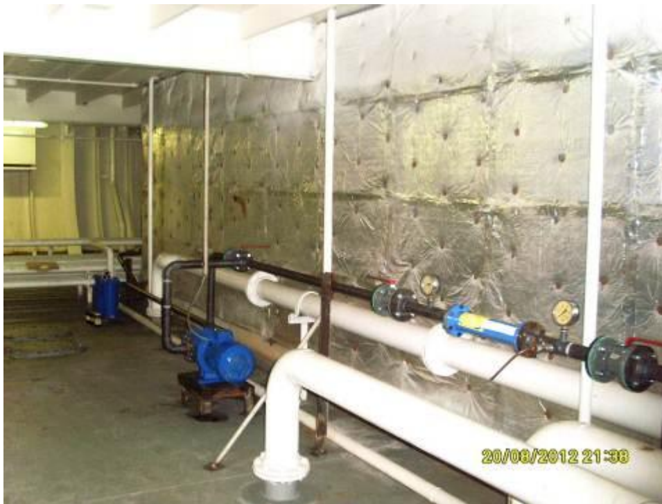
Module TRGA assembled on the settling tank
